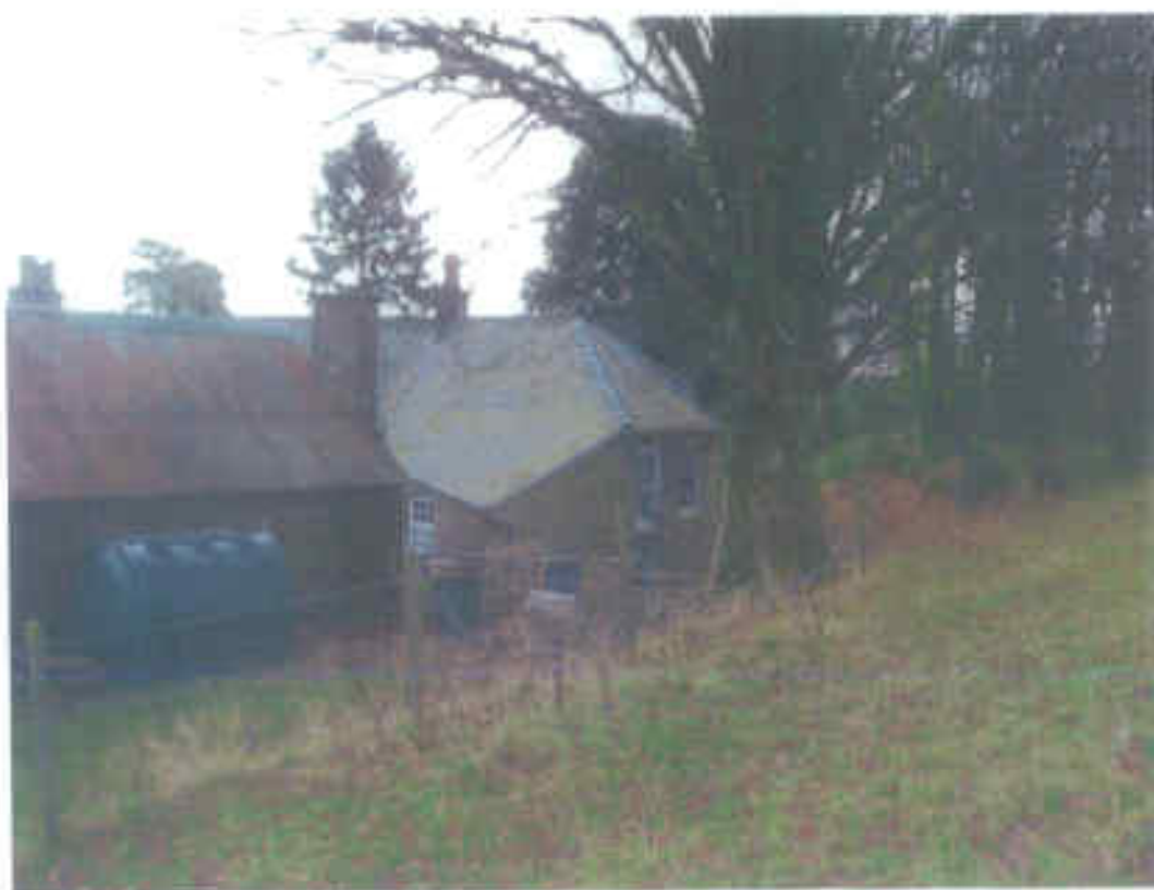
Fencing obstructing access into Tyle Gwyn Farm
